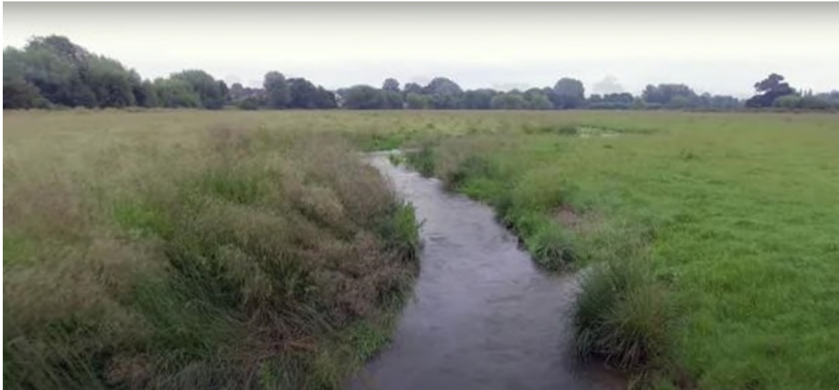
Figure 2. Example of a bypass channel designed to replicate a natural channel, River Great Ouse, Stony Stratford.
