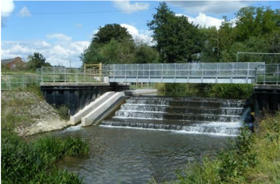
Figure 4. Example of a technical fish pass and eel pass (left hand side of weir), River Brit, Gundry's weir
