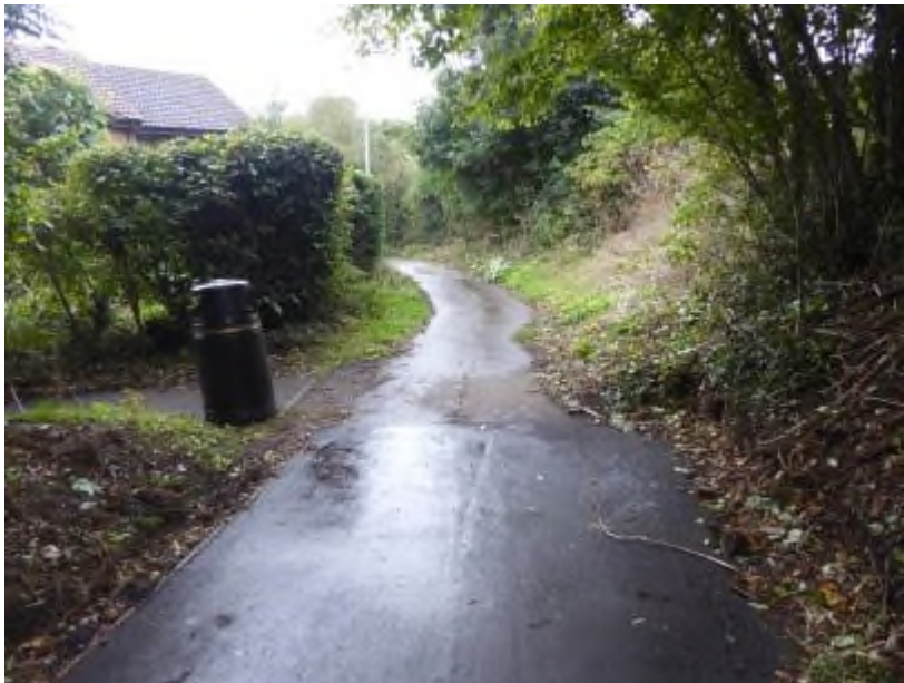
Section patched in 2019 leading into original tarmac surface
