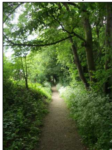
Crushed concrete Byway surface in wood
