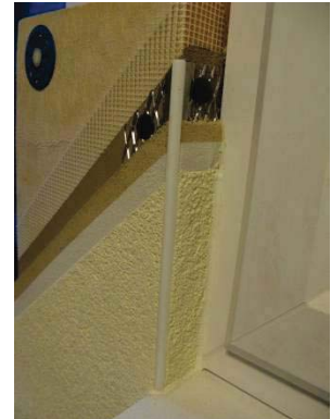
Cross-section of external wall insulation (credit: BioRegional)
