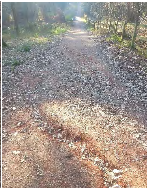
Fig 14 – Water damaged path
