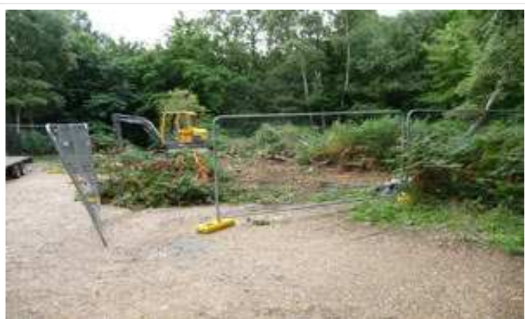
Broxbourne & Bencroft Woods car park refurbishment 2013-08 002
