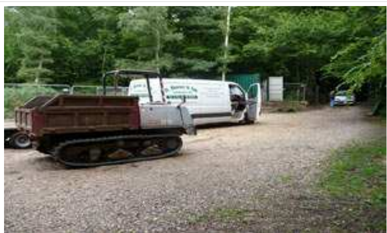
Broxbourne & Bencroft Woods car park refurbishment 2013-08 003
