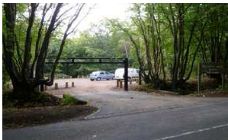
Broxbourne & Bencroft Woods car park refurbishment 2013-10 001
