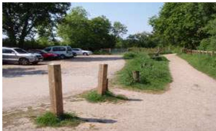
Broxbourne & Bencroft Woods car park refurbishment 2013-08 004
