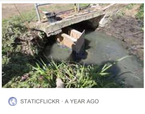
Wooden shuttering being installed to cast the concrete bridge support
