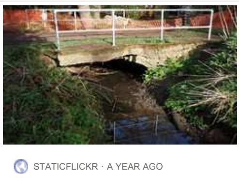
Bridge before repair works, lots of the bricks have become dislodged due to a large tree root
