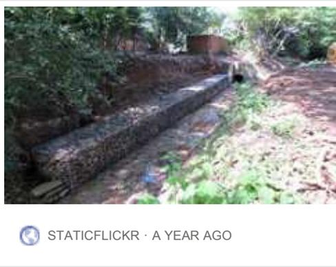
Row of gabion baskets installed to protect the bank edge from erosion
