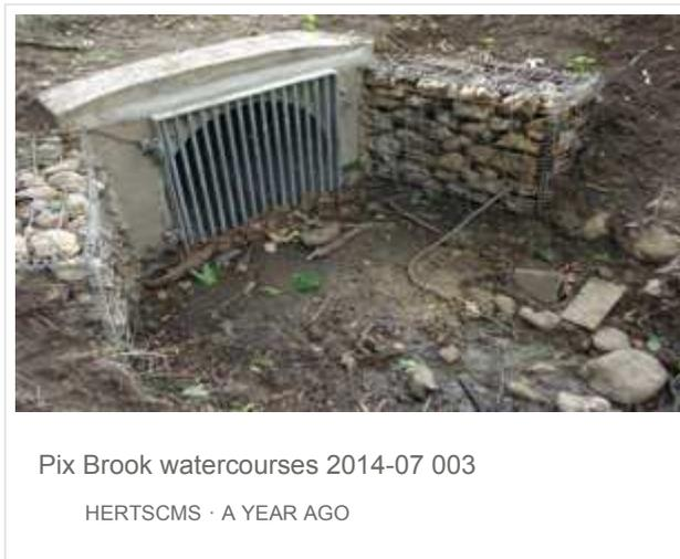
Trash screen to stop rubbish and debris from getting washed into Project D
