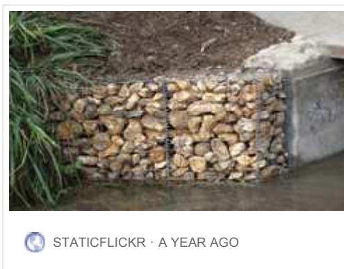
Gabion baskets and stone used to hide the concrete
