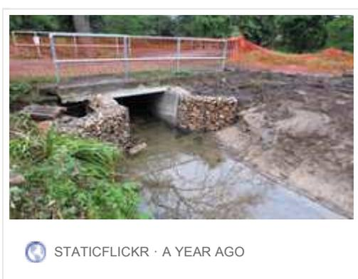
Gabion baskets installed both sides of the bridge to help funnel the water through the pipe
