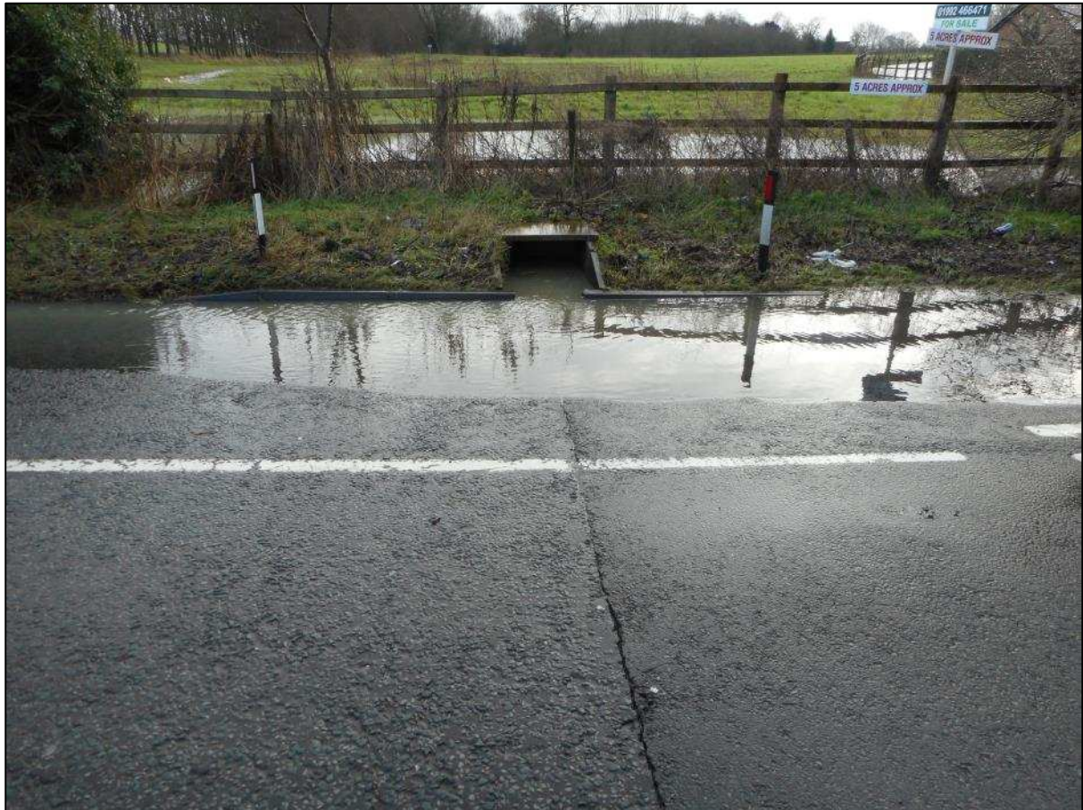
Figure 8 Water pooling on the highway, unable to discharge in the culverted watercourse, due to the culvert being at full capacity
