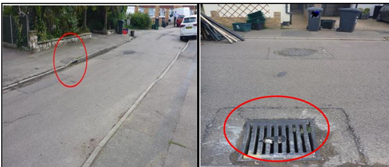
Figure 10: Origin of flooding to the highway in Admirals Walk investigation area
