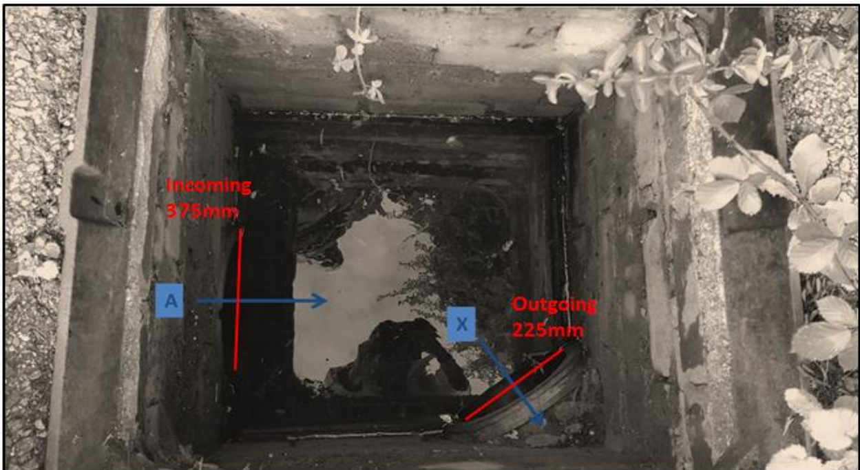
Figure 9: Incoming and outgoing pipes in manhole chamber 2 in Pallett Court
