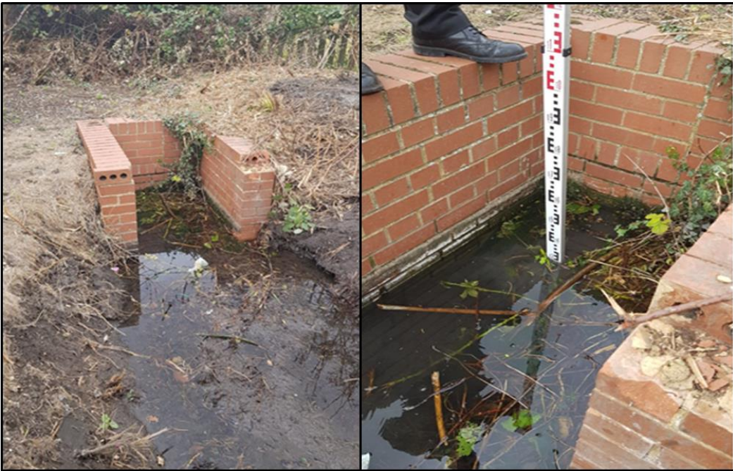
Figure 11: Outfall discharge point at the top of the ditch submerged
