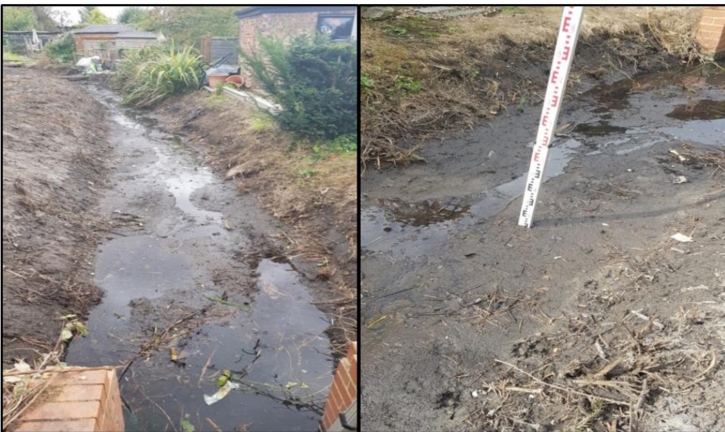
Figure 12: High levels of silt within the ditch
