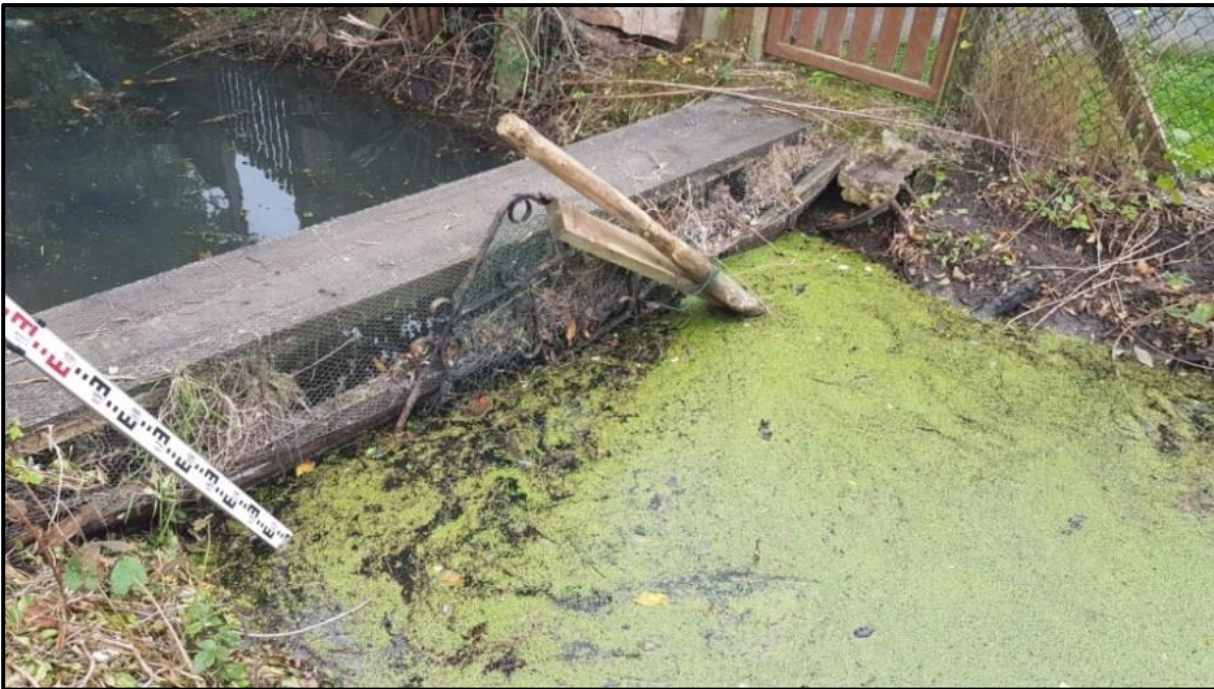
Figure 14: Existing blockages along the ditch
