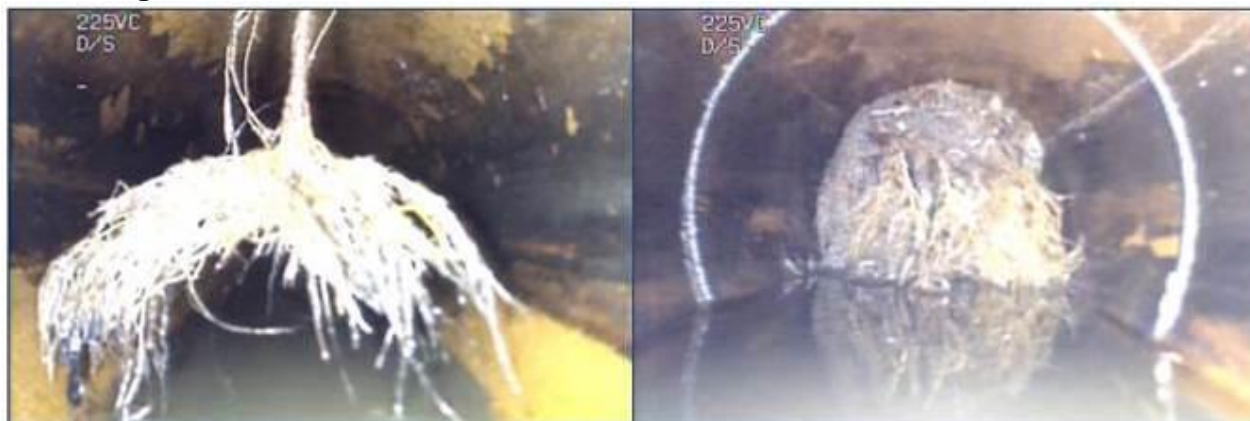
Figure 1: Images of failed CCTV Survey (25/11/2014). Root penetration visible in both images
