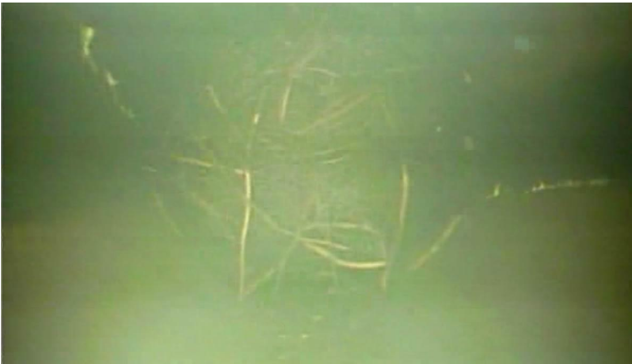
Figure 19 Collapse of soffit during the investigation
