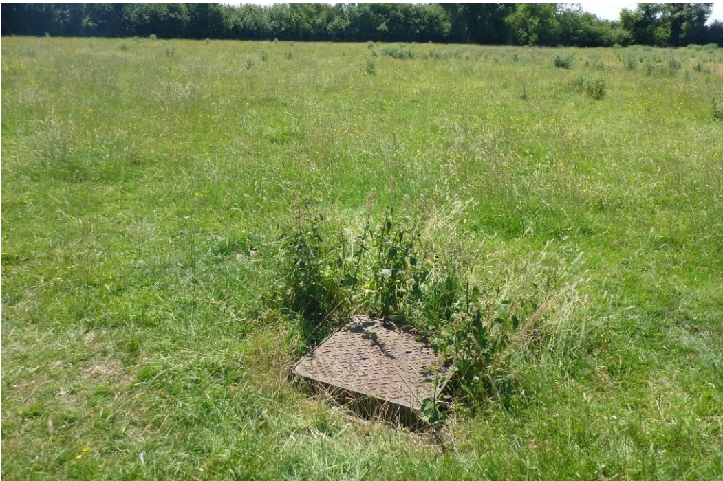
Figure 12 An example of a raised manhole through the farm near the pipe outlet
