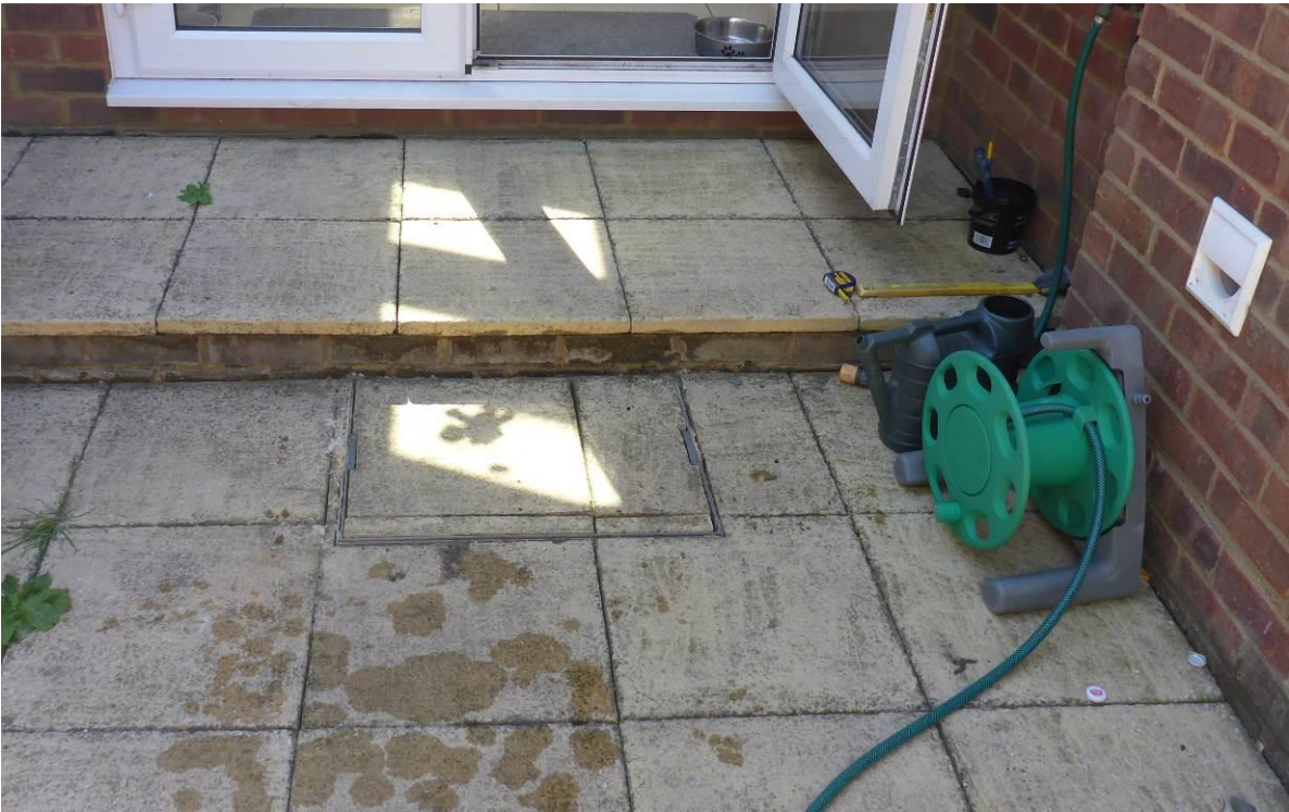
Figure 14 Manhole found upstream of flooded property
