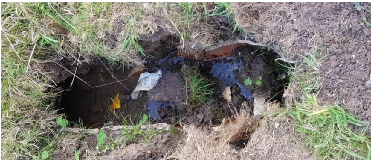
Figure 19 Collapse of soffit during the investigation
