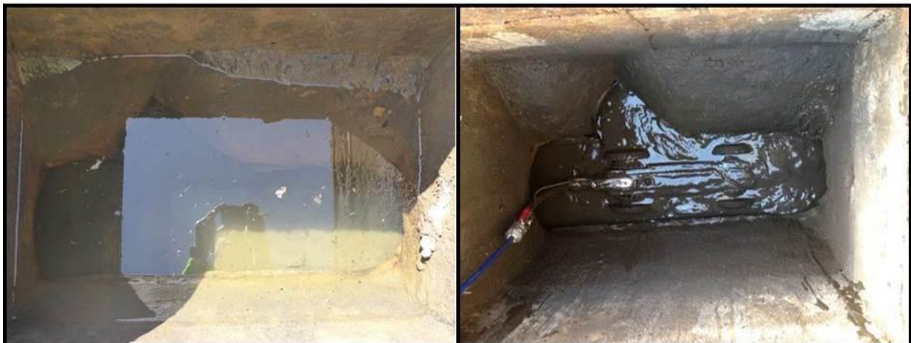
Figure 10 Standing water in the manhole chamber of the flooded property (Left image 2018, Right image 2014)
