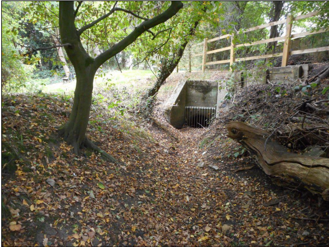
Figure 3 Ordinary watercourse culvert entrance
