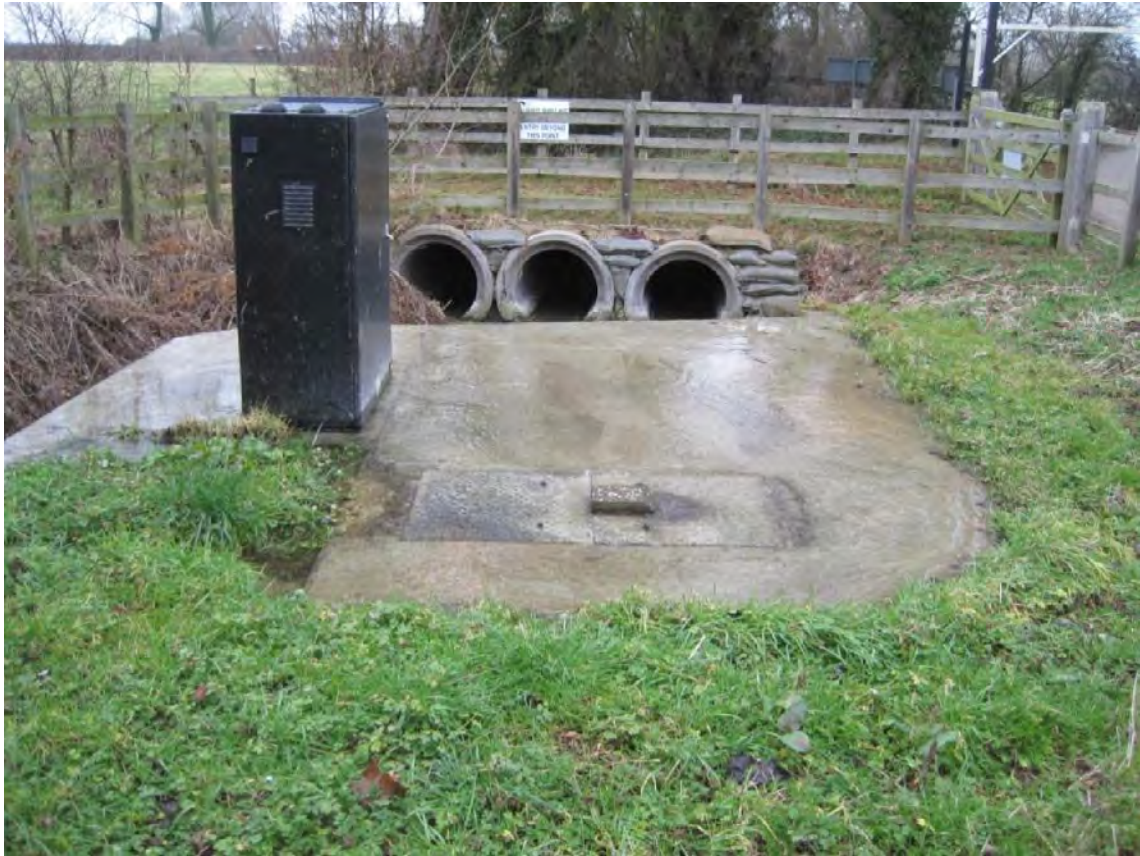
Wilstone Reservoir Syphon Outlet Chamber Looking Downstream
