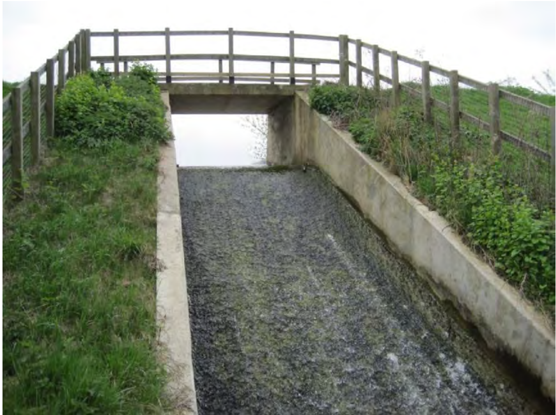
Wilstone Reservoir Overflow Weir
