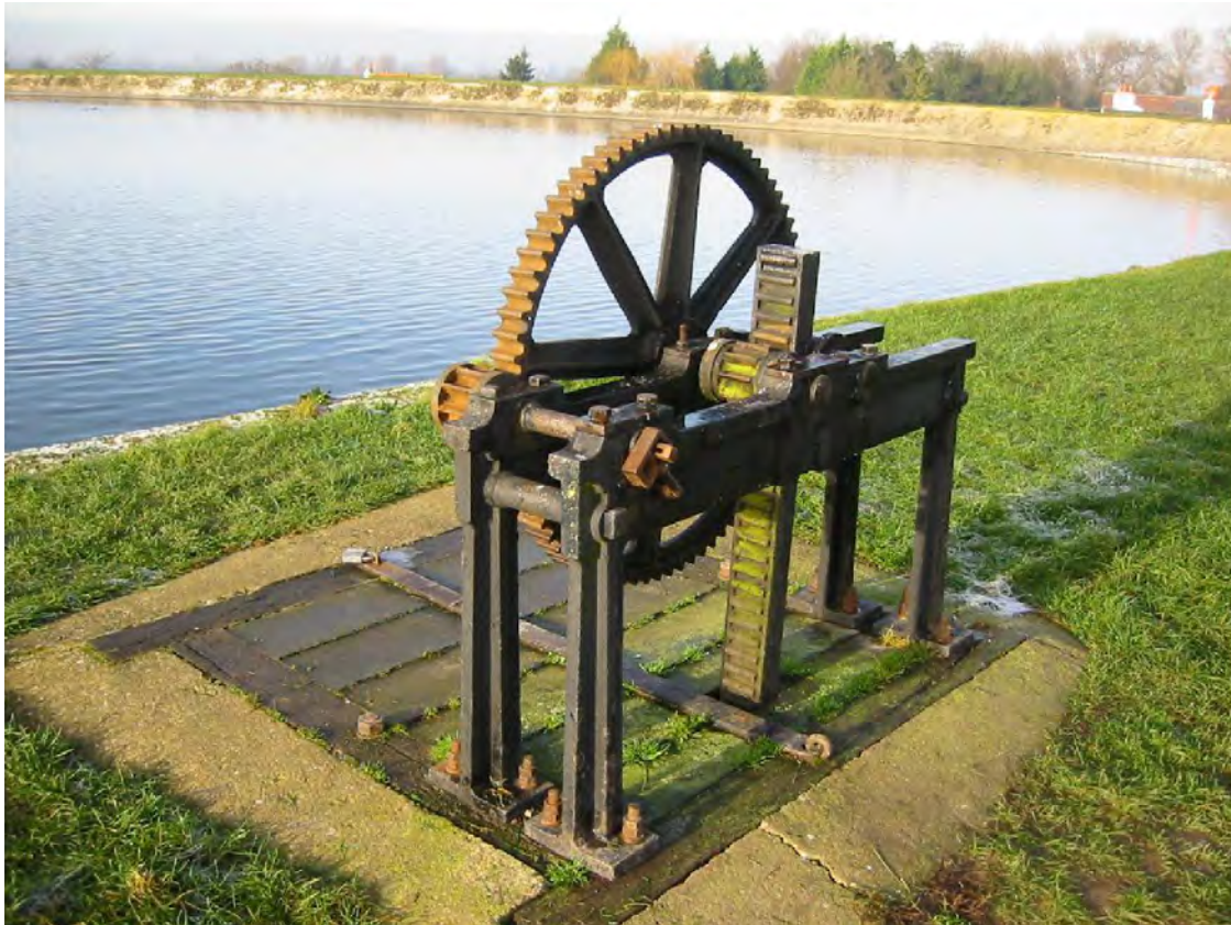
Startops Reservoir Outflow Sluice Gearing Discharges to Startops Feeder
