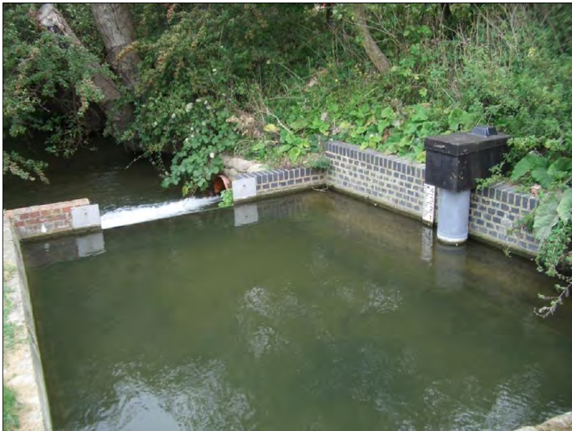
Startops (and Marsworth) Reservoir gravity outflow into Startops Feeder
