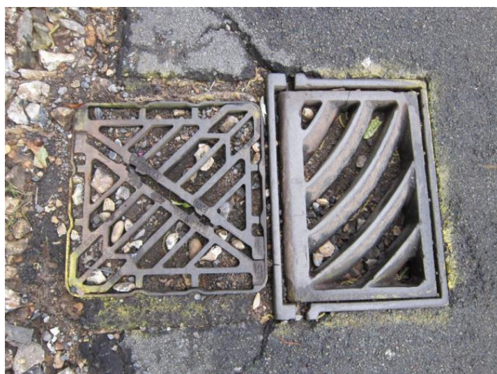
Figure 9: Blocked Gullies in Lybury Lane (Image taken following the storm event in February 2014)
