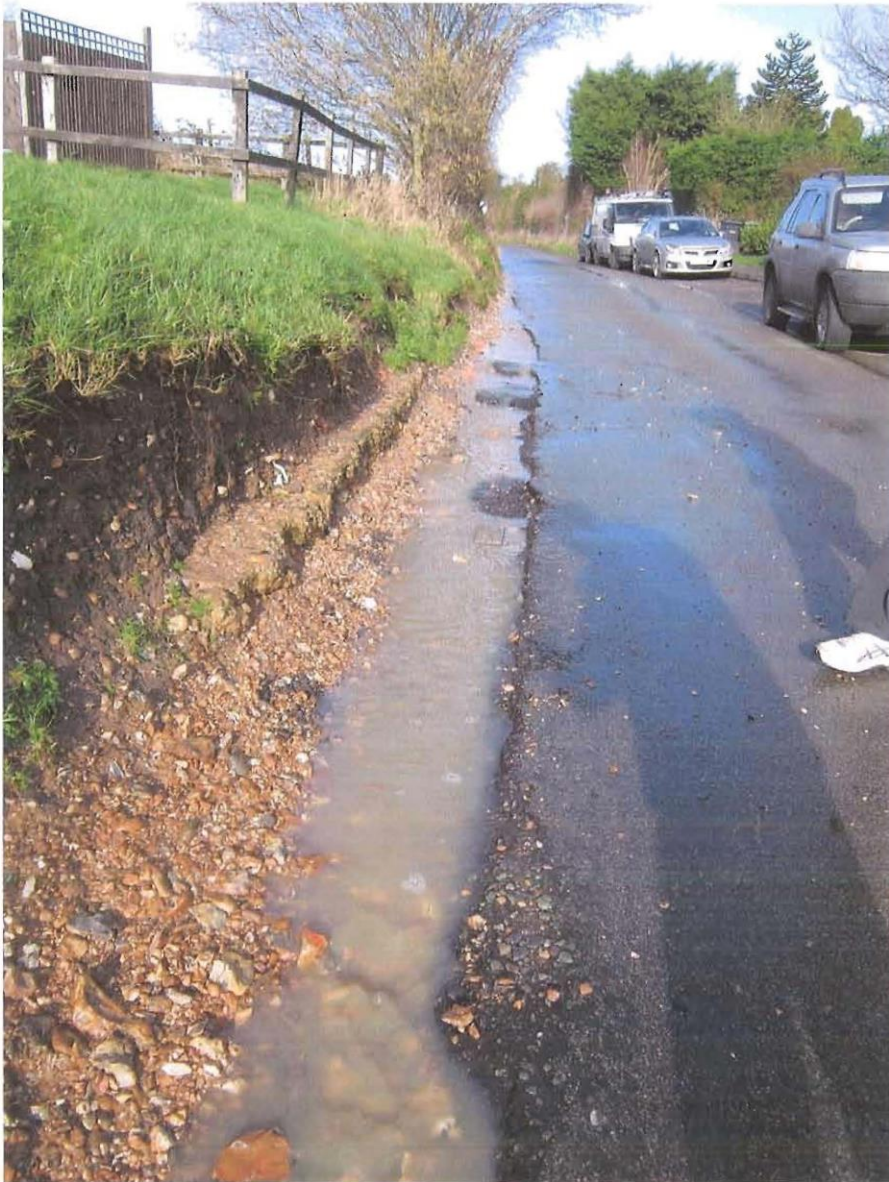
Top of Lybury Lane – Stream of water due to blocked drains further up the road. Note the erosion of the road. The drains have been blocked for several months which has caused this.
