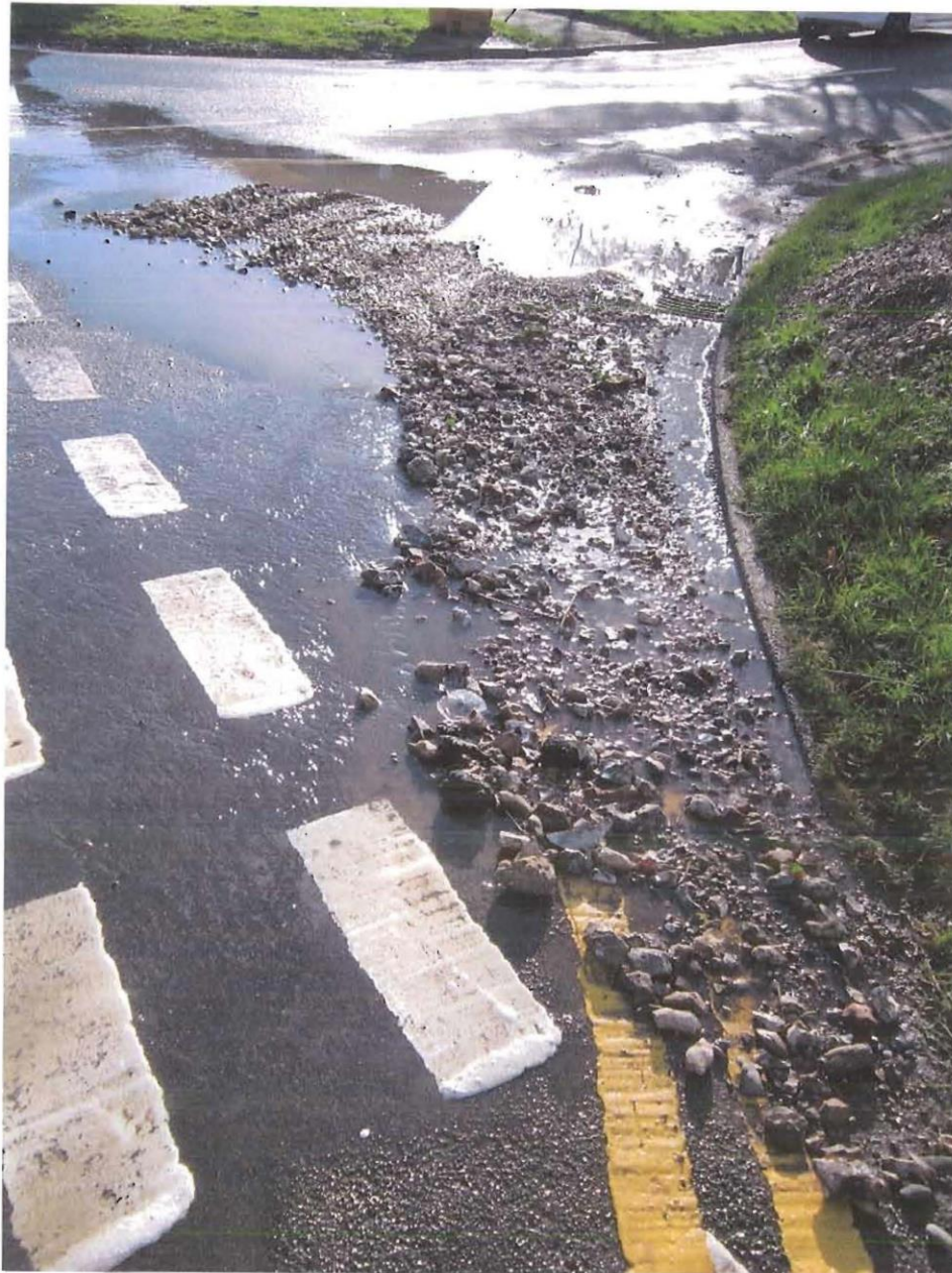
Top of Lybury lane – showing debris blocking drains.
