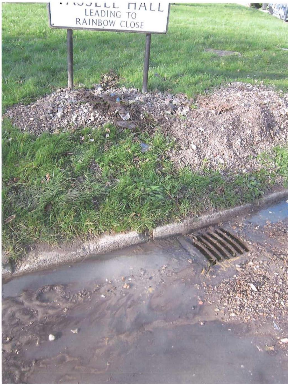
Top of Lybury Lane – Debris blocking drains – Note the amount of debris on the grassed area that has already been hand cleared from the tops of the drains by local residents.
