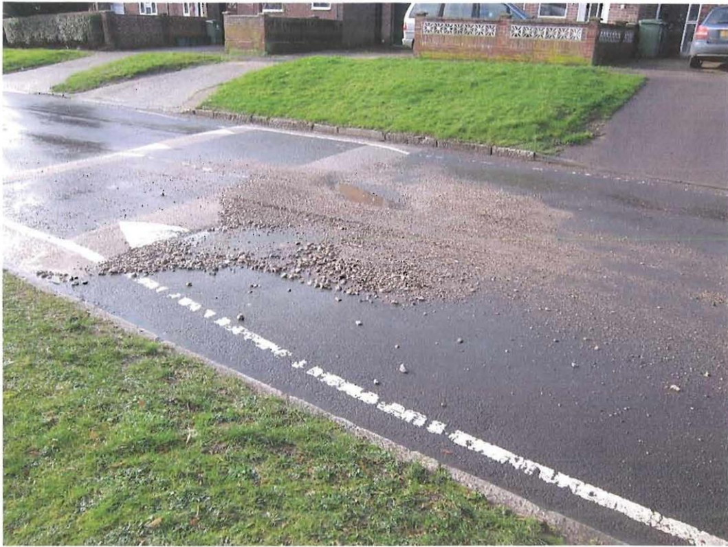
Midway down Lybury Lane – Debris swept by flood across whole road.
