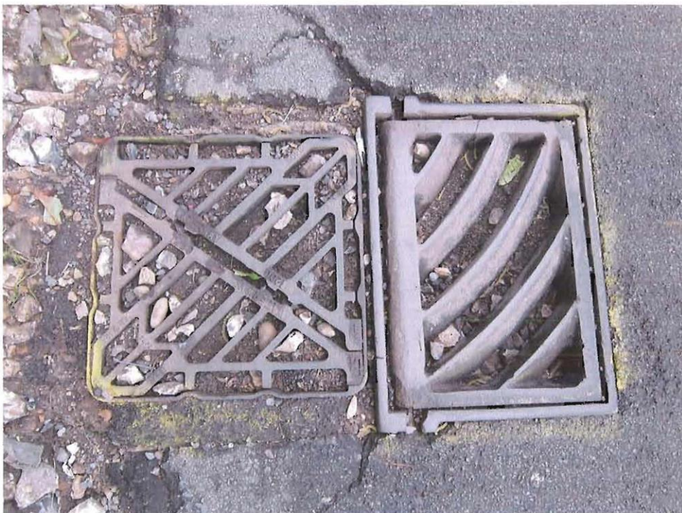
Top of Lybury Lane – Two blocked drains (photo taken 10/02/14).
