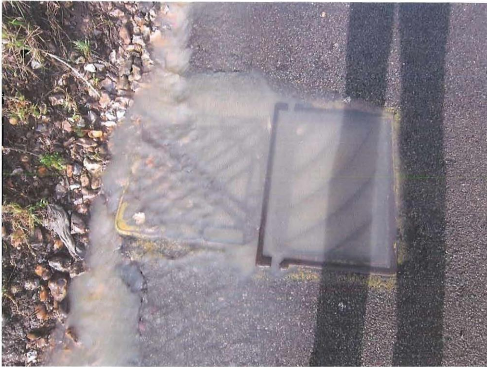
Top of Lybury Lane – Two blocked drains, completely full to the top with debris.
