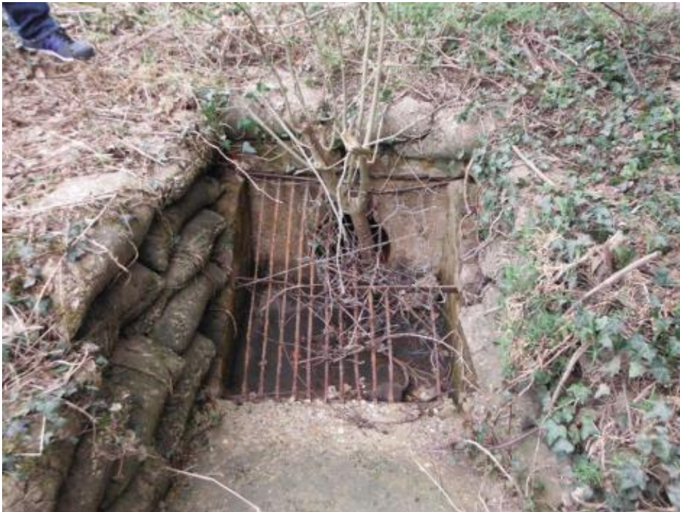
Figure 5 – Culvert at the junction with Robbery Bottom Lane
