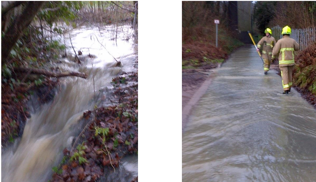
Figure 6 – Overflow from Robbery Bottom Lane culvert flowing west along the road
