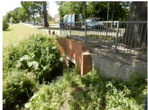
Figure 23: Culvert under Goff's Lane from nearby pond
