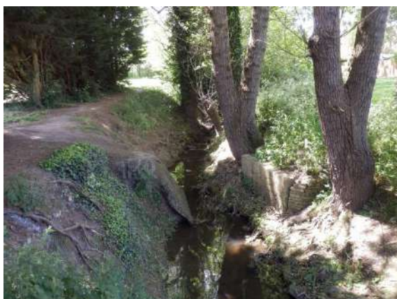
Figure 18: Rags Brook Upstream of Figure 17, channel is well incised; water level is approx. 1.5m – 2m below top of bank.
