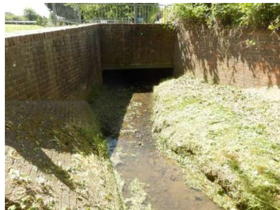
Figure 17: Culvert under Rosedale Way Near to Fourfields Quantum Care Home. Maintenance work was being conducted on the day of the site visit, grass cutting, channel debris removal etc.
