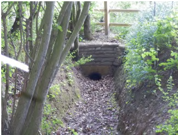
Figure 11: Headwall and culvert under railway
