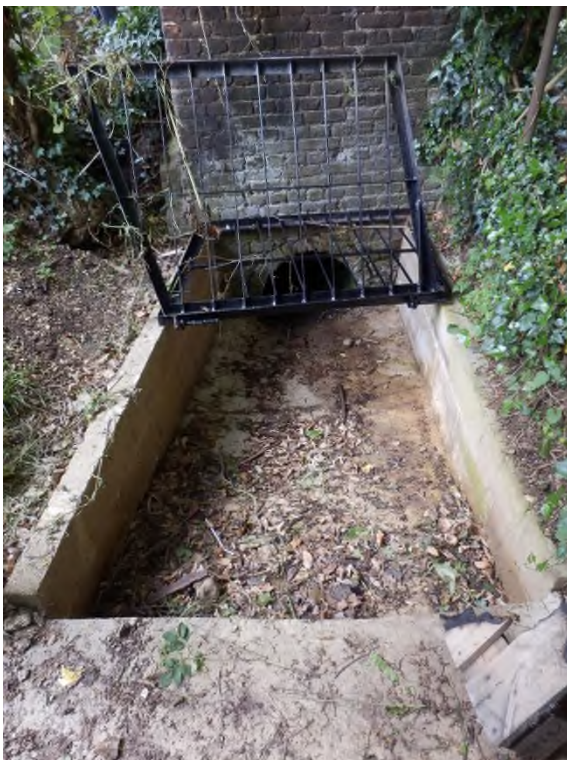
Figure 24: Brick culvert and screen
