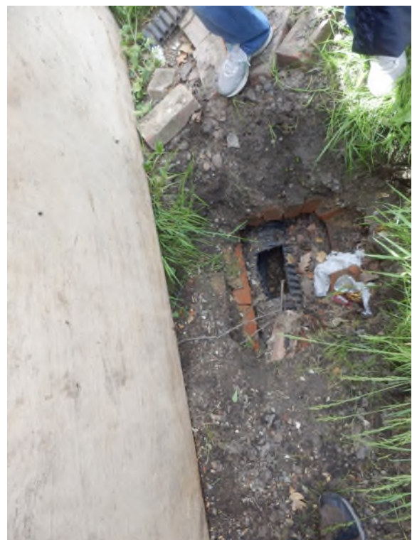
Figure 25: Brick culvert and screen
