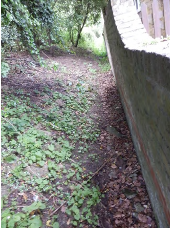
Figure 22: Ditch to the side of Hadham Cross Fire Station
