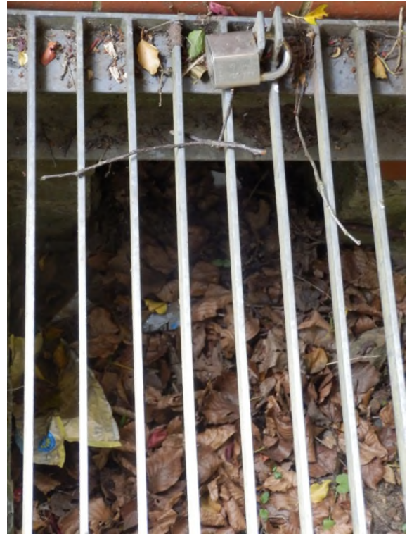
Figure 23: Culvert/ditch contains lots of detritus Vegetation and detritus has fallen/passed through the screen.
