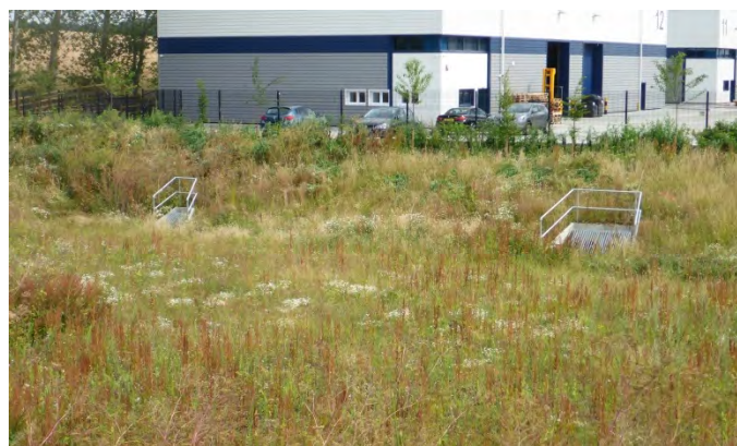
SuDS attenuation basin, Bourne End, Dacorum
