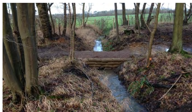
Structure with culvert across an ordinary watercourse, Oxhey Woods
