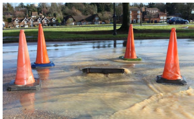
Surcharged manhole (the sewer system has reached its capacity and water escapes), Harpenden
