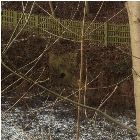
Figure 19: Outfall into A1(M) retention feature
