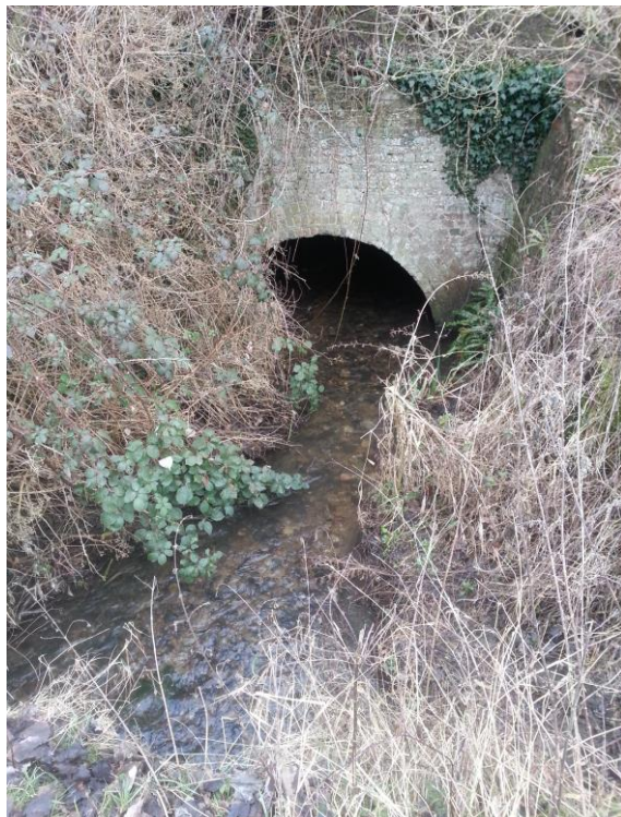
Figure 8: Culvert under railway track
