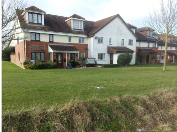
Figure 12: Existing Residential Properties
