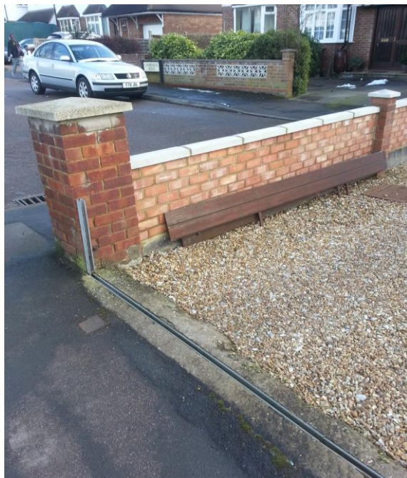
Figure 22: Property located along the A505 with protection measures
