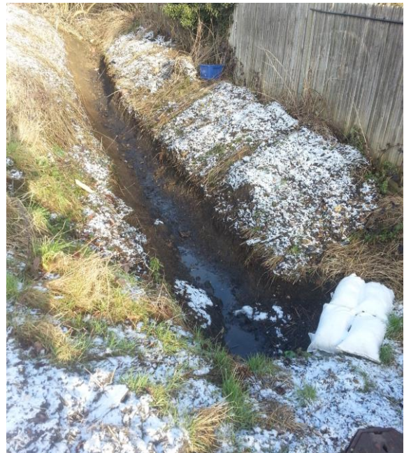
Figure 20: Recent flood mitigation works
