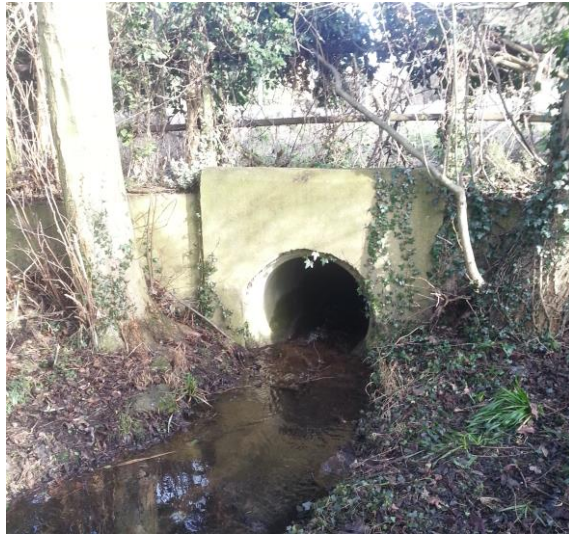
Figure 6: Culvert under the A602, looking south
