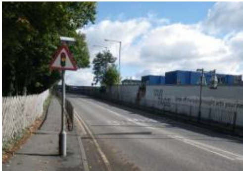
Figure 2 – Allum Lane Looking east across railway
