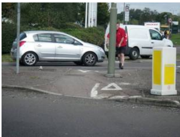
Figure 4 - Splitter island on A411 Barnet Lane (west) arm. Obstruction across the cycle path. Only a small area for cyclists/pedestrians to wait.
