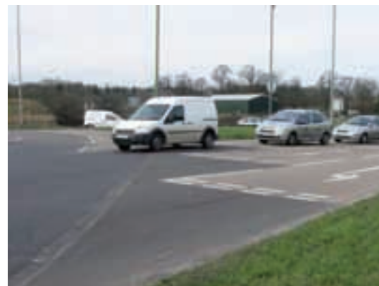
Photograph 1: Staggered stop lines on A10 (North) approach to junction
