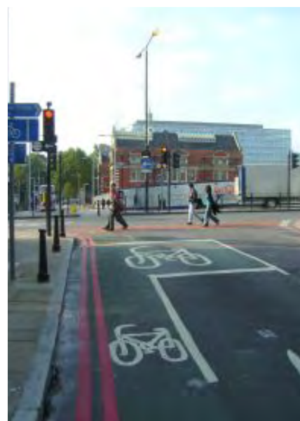
Examples of advanced stop lines for cyclists – priority is given to cyclists in the 'box' so that they may gain an advantage over stationary traffic at a signalised junction. This also helps provide a safer road position for cyclists wishing to turn left or right at the signals.
