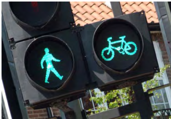
Example of a Toucan crossing – This facility will be more suitable for cyclists wishing to cross Nightingale Road and forms an important link as part of the proposed cycle route 4
