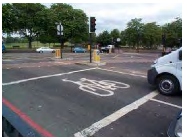
Examples of advanced stop lines for cyclists – priority is given to cyclists in the 'box' so that they may gain an advantage over stationary traffic at a signalised junction. This also helps provide a safer road position for cyclists wishing to turn left or right at the signals.
