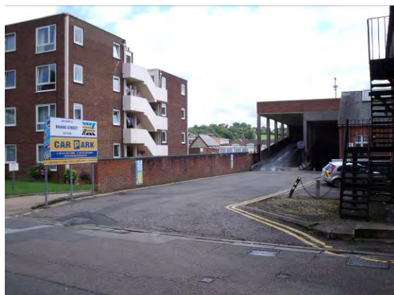
Brand Street car park – The introduction of real time information would update motorists as to the availability of parking spaces in Town Centre car parks
