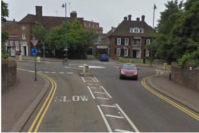
Plate 1 – Southern end of Bridge Road showing bollard pinch point and roundabout with Station Way
