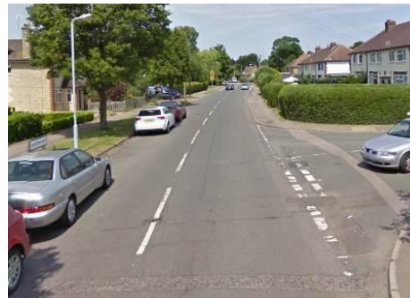
Plate 2 – Weston Way northbound, junction with Park Drive on the right
