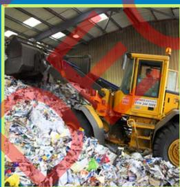
The tipping floor at a MRF. Incoming materials are received and stored here prior to processing. Tipping floors should be covered to prevent leachate into groundwater and contamination of water supply.
