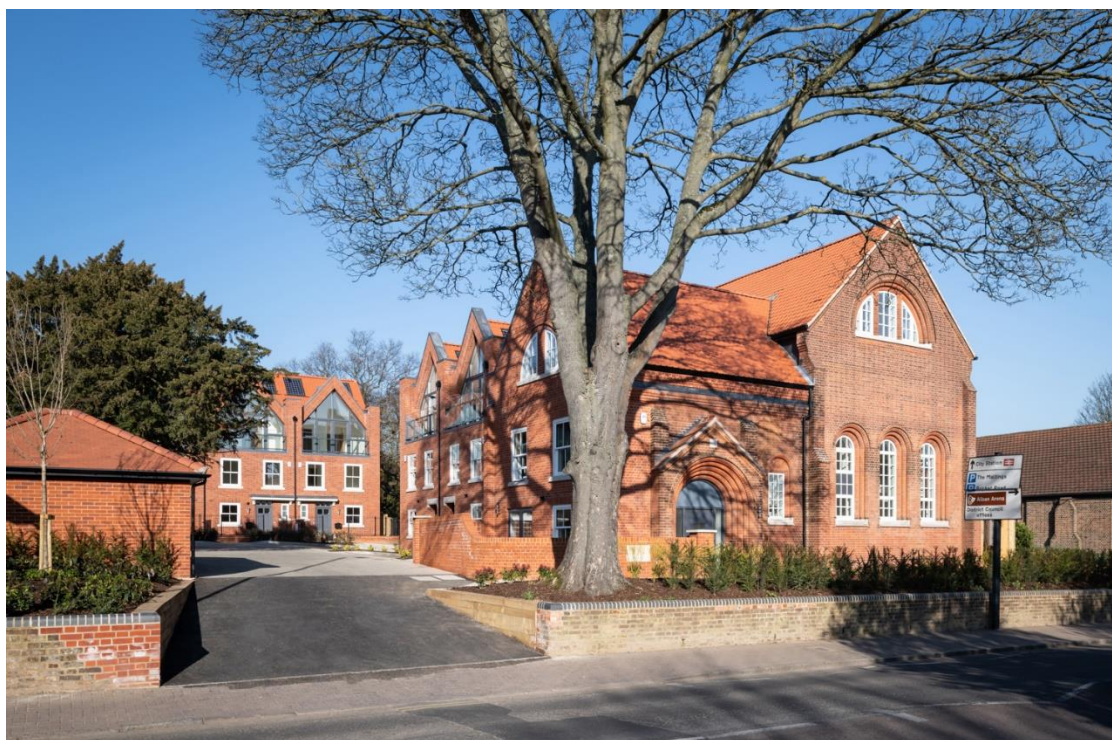
© Morgan Sindall Construction
